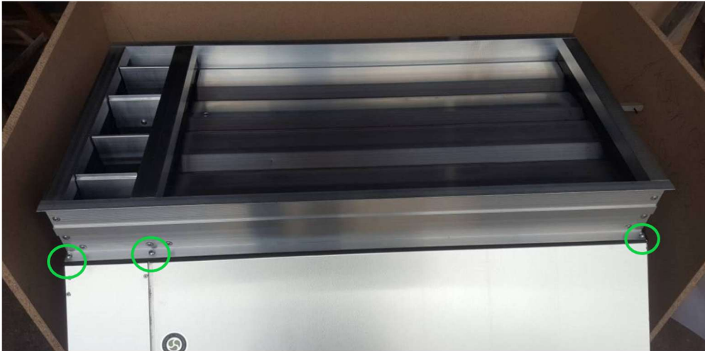
Self tapping screws in each corner of exchanger and bypass
