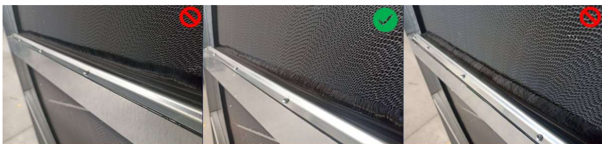
Positioning of central (diameter) seals
